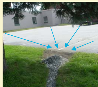
Estimating the stormwater that runs off streets, sidewalks, and parking lots can be tricky. It is best to visit the impervious area during a rain event to clearly see the extent of the drainage area.
