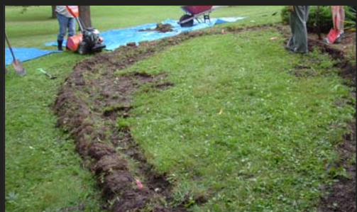
Build the berm with sod
