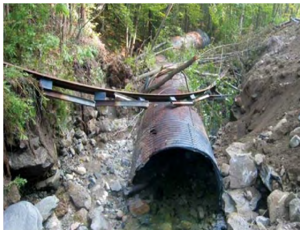
Road failure at a 3-m culvert placed within a 6-m bankfull width stream, GMNF
