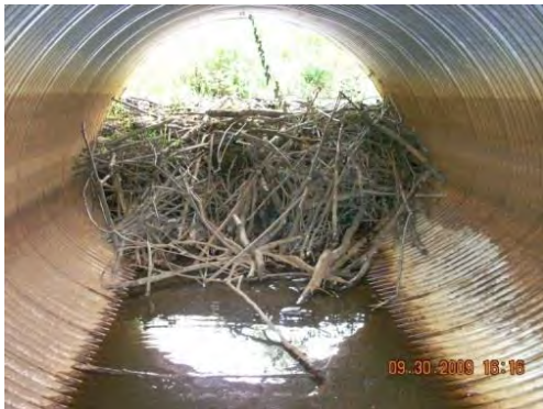
Undersized culverts, which constrict flow, are almost irresistible to beavers. Source: www.martinezbeavers.org/wordpress
