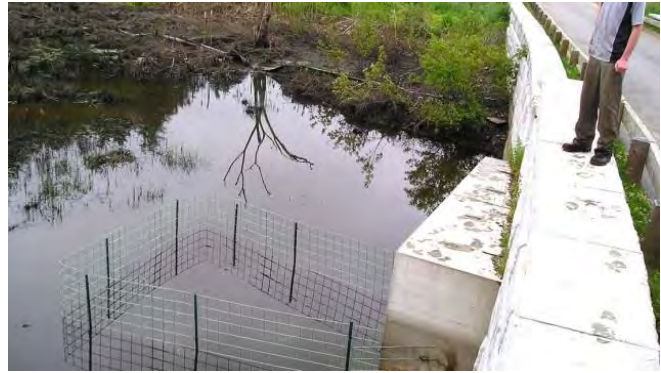
Culvert fences are the most commonly used beaver device by the Forest Service, however they may block fish passage. USFS concludes that the best solution is culvert replacement. Source: www.beaversolutions.com
