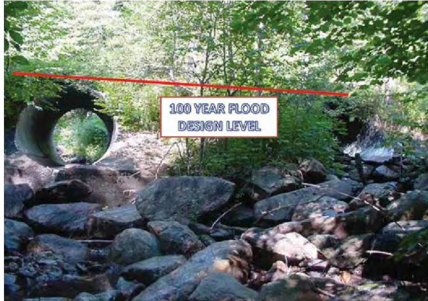
Double-barrel hydraulically designed culvert on Jenny Coolidge Brook, Green Mountain National Forest, VT
