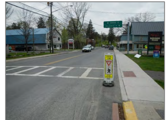
Curb extensions and more visible warning signs would improve safety at the trail crossing on Main St.
