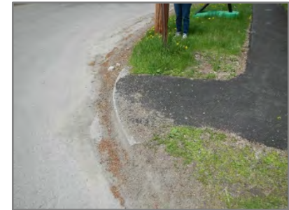
This curb (on Park Street) lacks a ramp and warning strip.
