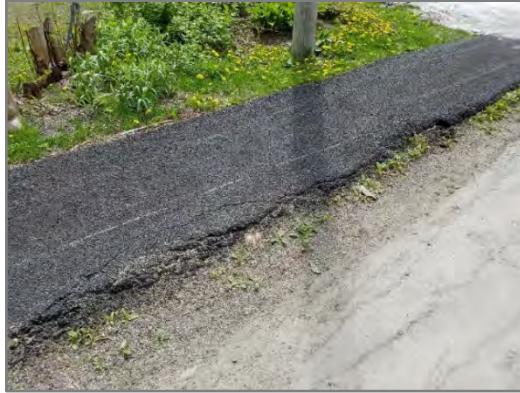
Asphalt sidewalks often ravel (crack and break off) along the edge, reducing the useable width.
