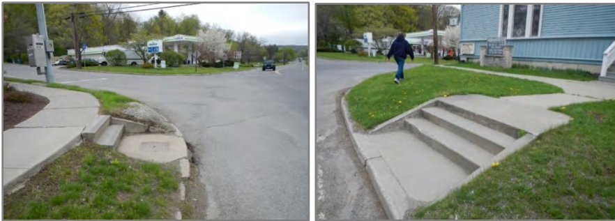
The Main/Maple intersection lacks curb ramps, crosswalks, and pedestrian signals.
