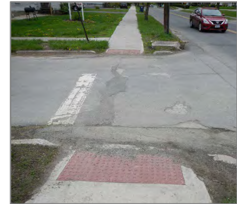
ADA compliant ramps have detectable warning strips (like these on Main Street) to warn visually impaired persons of the transition from sidewalk to street.
